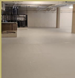
03 BASEMENT/ CELLAR WP
